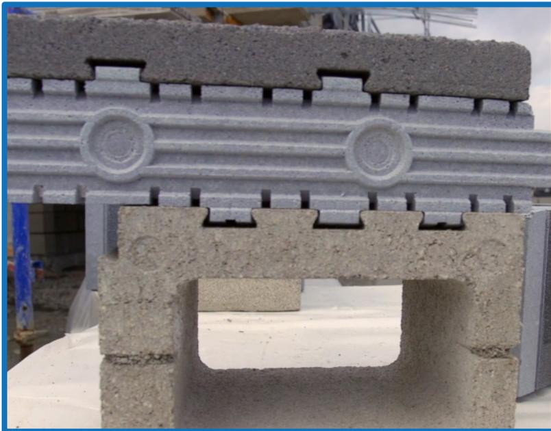
+ Oldcastle® and Plymouth Foam worked together to develop the InsulTech™ insulation insert system. The innovative product line is a new commercial insulated concrete masonry system. Plymouth Foam developed the molded Neopor™ insulation piece between the structural masonry unit and the thin veneer face.
